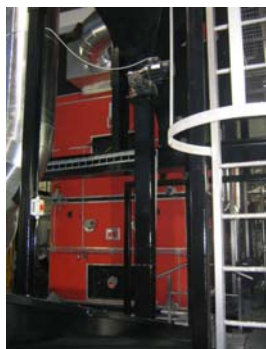
Watercooled grate system
